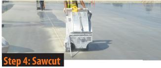
• Sawcut the joint (1/4 of slab thickness) as soon as the concrete will support the saw and operator.
